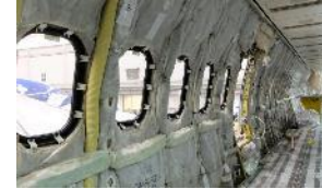
Complete Interior Removal / Installation
